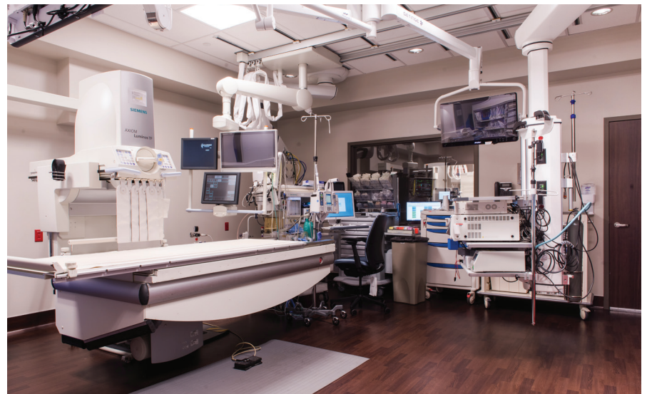
The new GI lab features two advanced fluoroscopy procedure rooms with new equipment in a high-tech setting.
